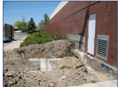
The footings for the school's new entrance! (Photo taken April 28, 2006).
